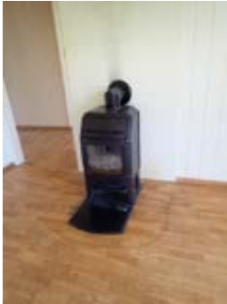
Ovn for fast brensel over stålplate
