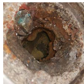
Eldre jern / soil sluk uten klemring.
