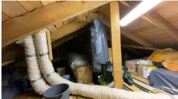
Begrenset adgang for kontroll.
