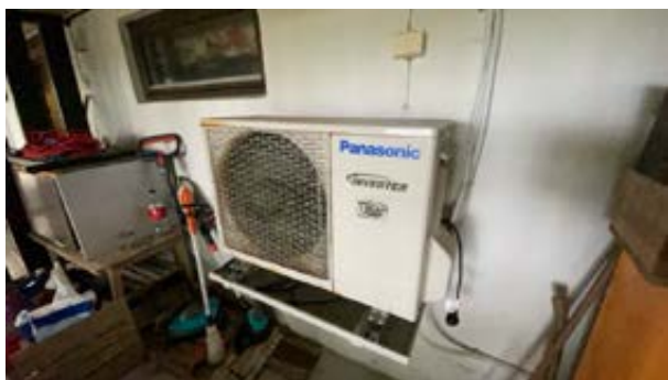
Utedel varmepumpe.
