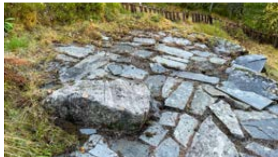
Steinplatting, ujevnheter etc
