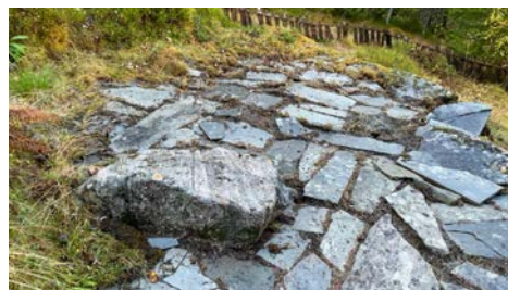
Steinplatting, ujevnheter etc
