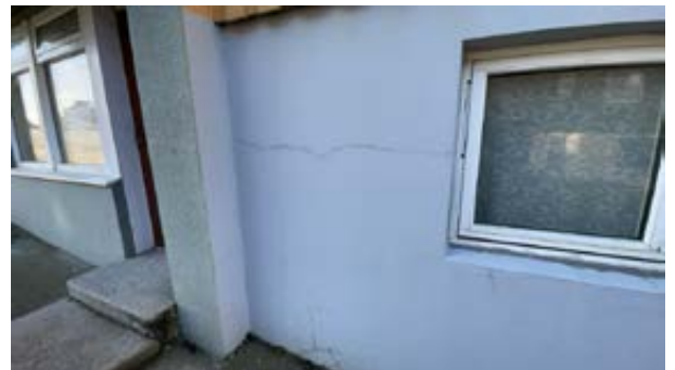
Mindre riss/sprekker
