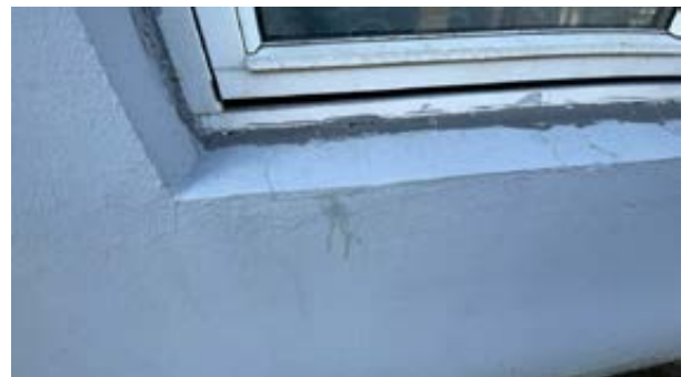
Mindre riss/sprekker.
