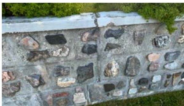
Stedvis riss/sprekker.
