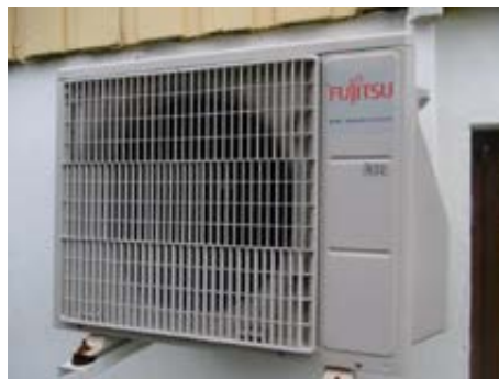
Varmepumpe ute del.
