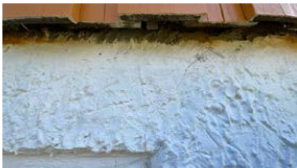
Mindre riss/sprekker.
