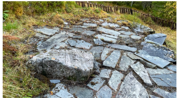
Steinplatting, ujevnheter etc
