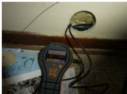
Hulltaking utforet vegg under terreng
