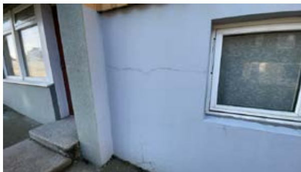
Mindre riss/sprekker
