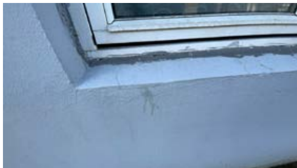
Mindre riss/sprekker.
