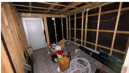
Rom under renovering
