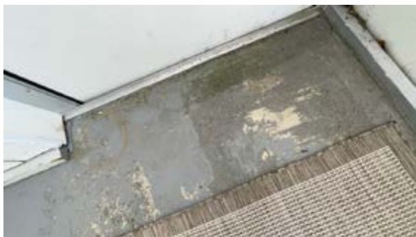
Slitt betongplate.
