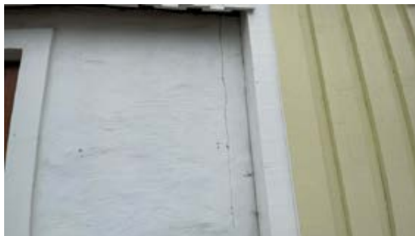
Mindre riss/sprekker.
