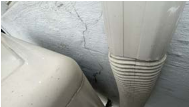
Mindre riss/sprekker.
