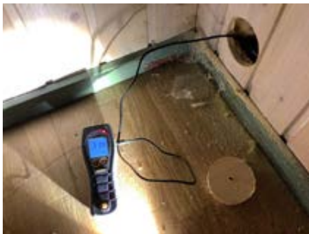
Hulltaking under hall.
