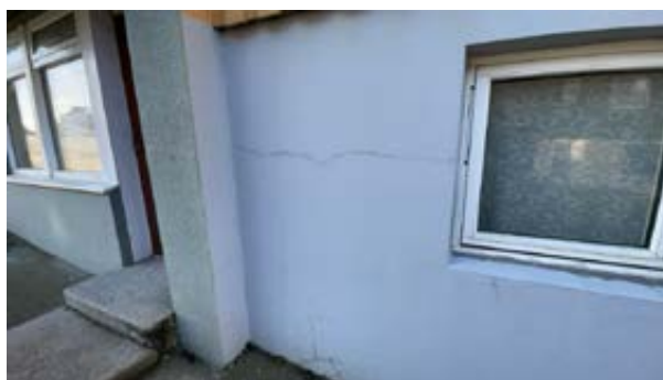
Mindre riss/sprekker
