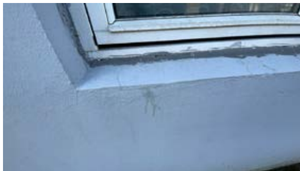
Mindre riss/sprekker.
